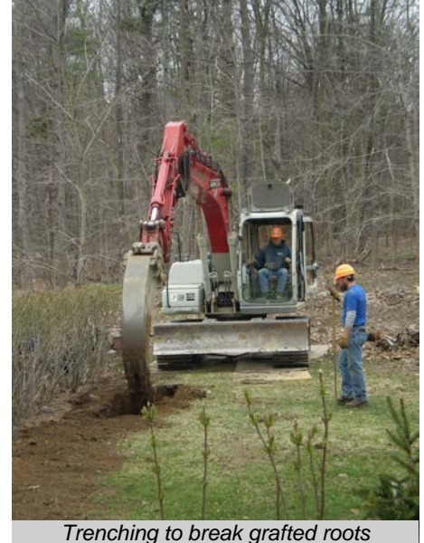
Trenching to break grafted roots
